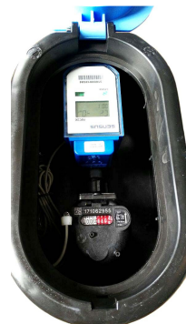
Surface or Wall mount with Sensus 220C meter
